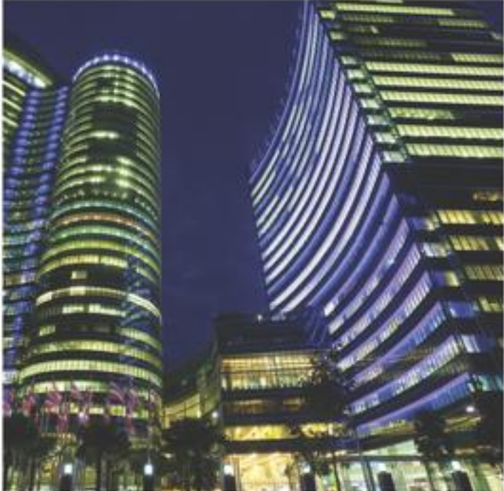
Image Source: www.energycomplex.co.th
